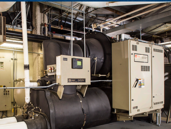
The demand limiting feature on chillers was enabled to limit chiller capacity during peak energy use periods.
